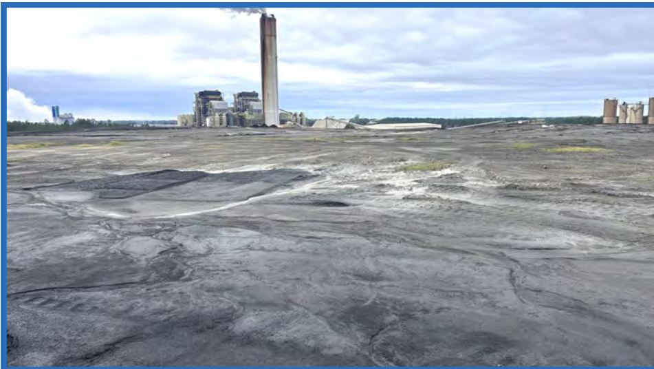
Top of Waste in Increment 1, Looking Southwest
