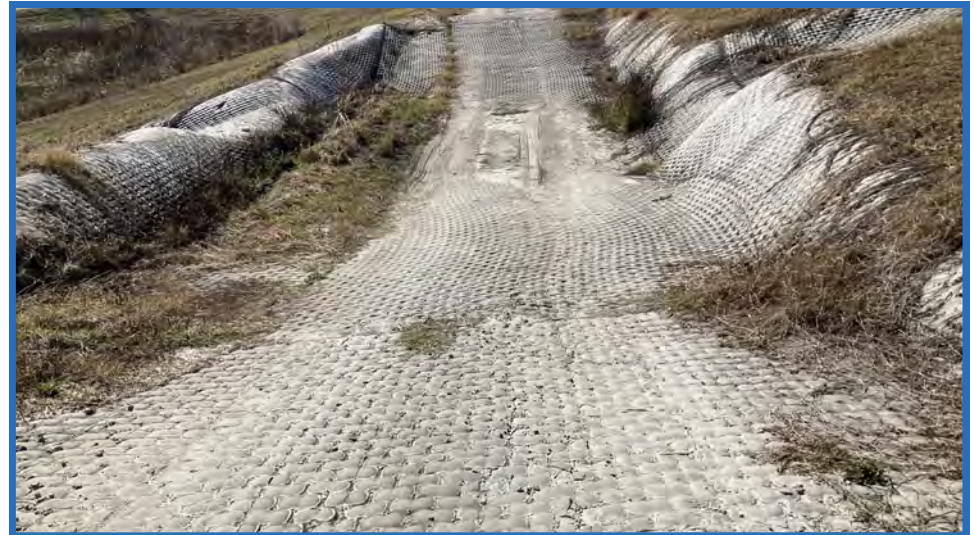
Fabriform-Lined Flume on Southern Part of Eastern Slope of Containment Dike for Stage I and Perimeter Road, Looking South
