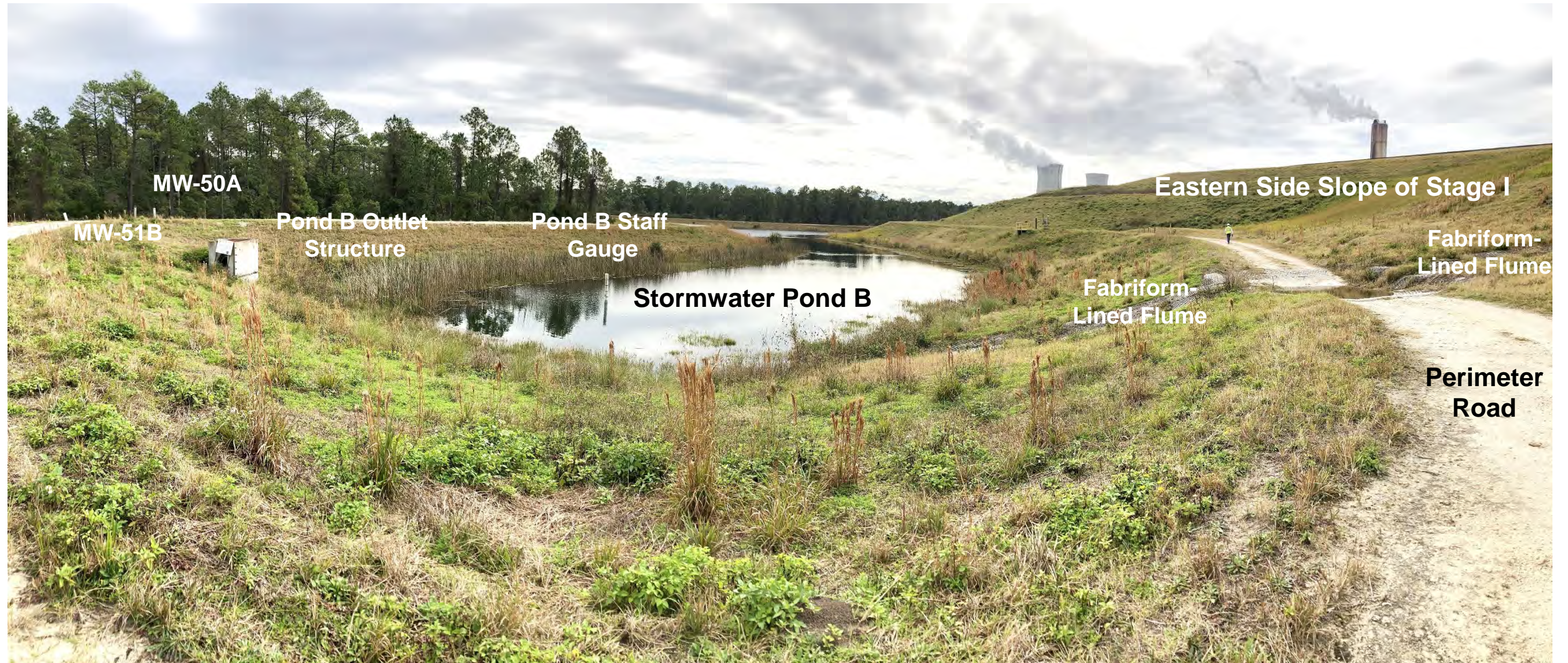
Increment 1, Stage I Eastern Side Slope and Containment Dike, Looking South from Road at Northern End of Stormwater Pond B
