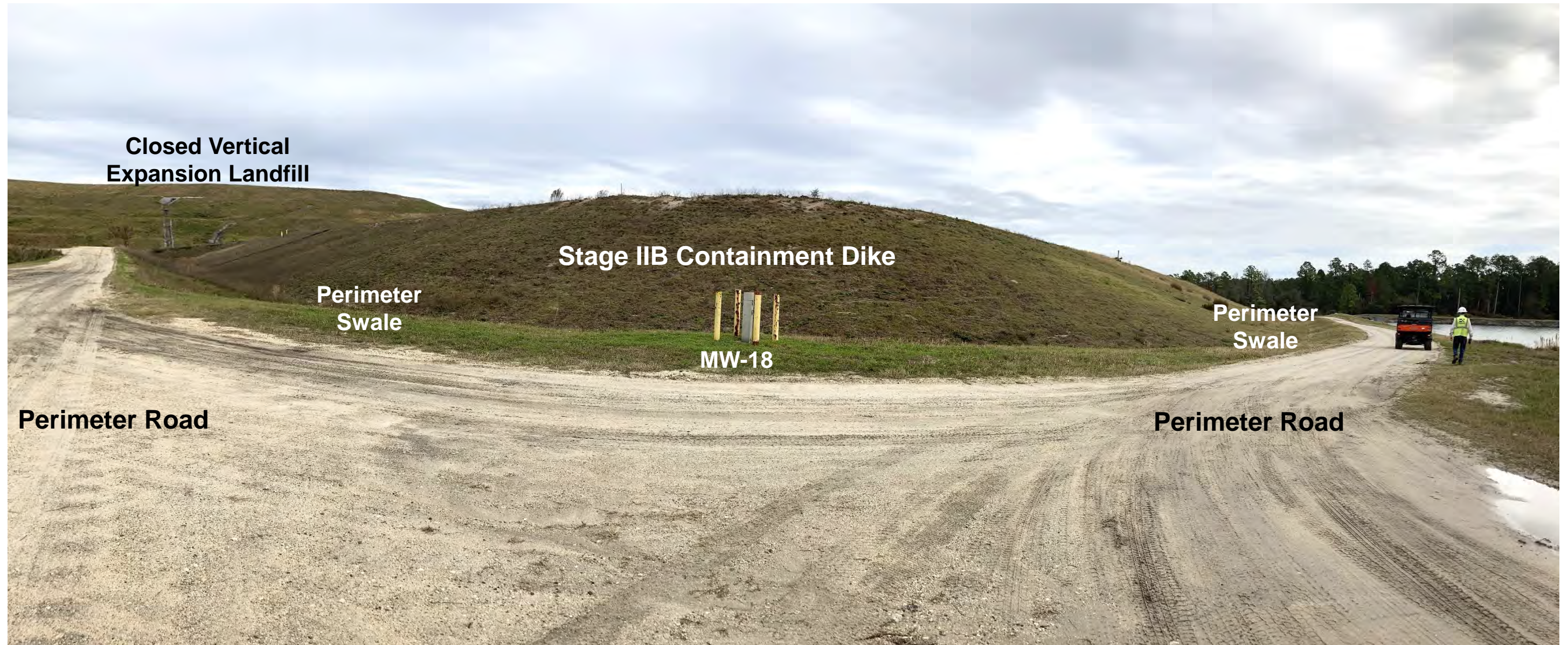
Panorama Along Perimeter Road and Swale, Looking Northeast from Perimeter Road at Southwestern Corner of Stage IIB Containment Dike
