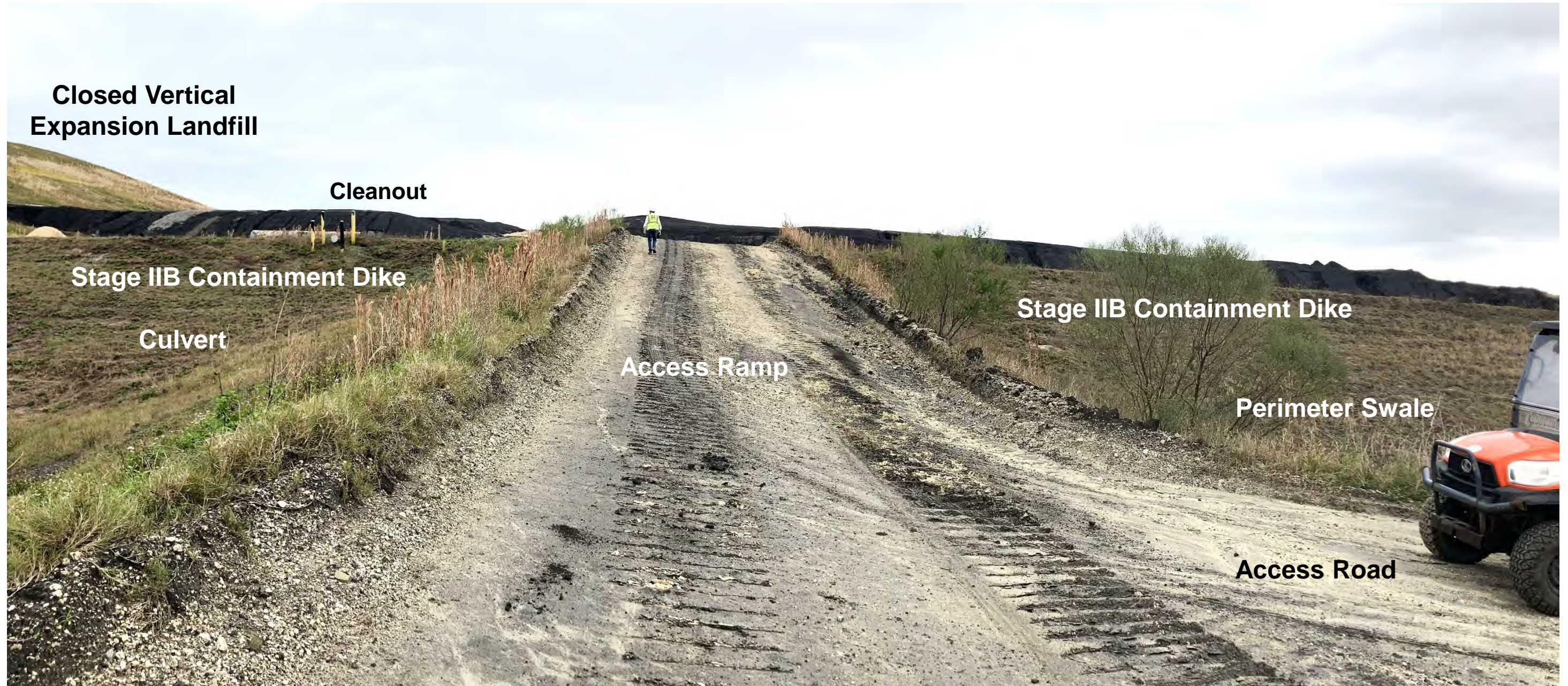
Access Ramp to Stage IIB, Looking East Toward Increment 1 Buildout
