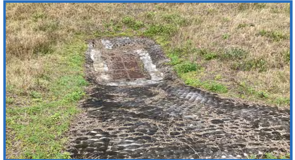
Stormwater Inlet in Southeastern Corner of Increment 1
