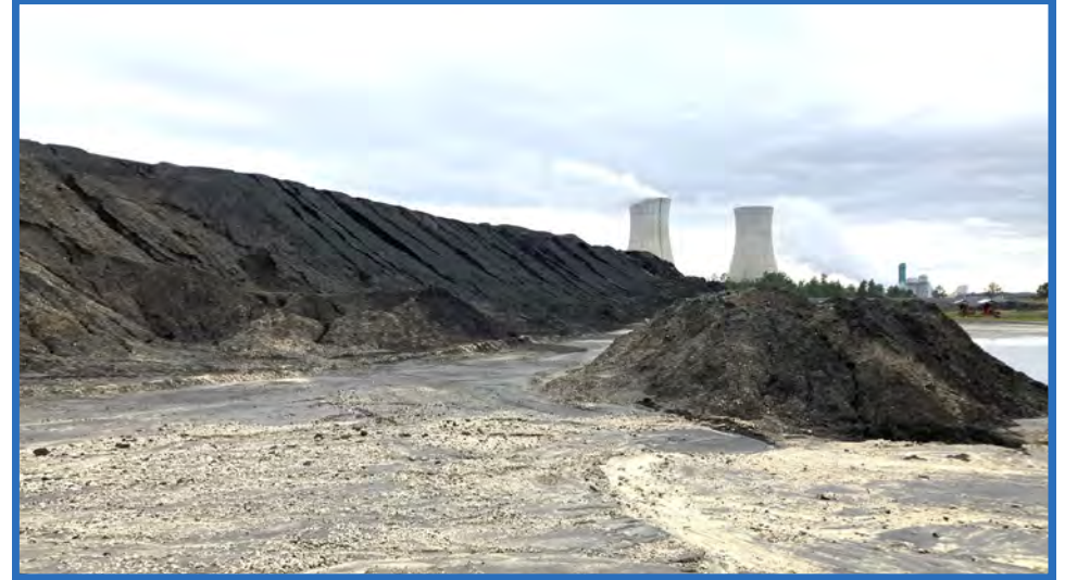
Access Ramp through Stage IIB, Looking Southeast
