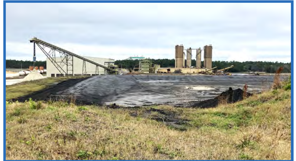
Pozzocrete Dike in Southern Part of Stage IIB, Looking West
