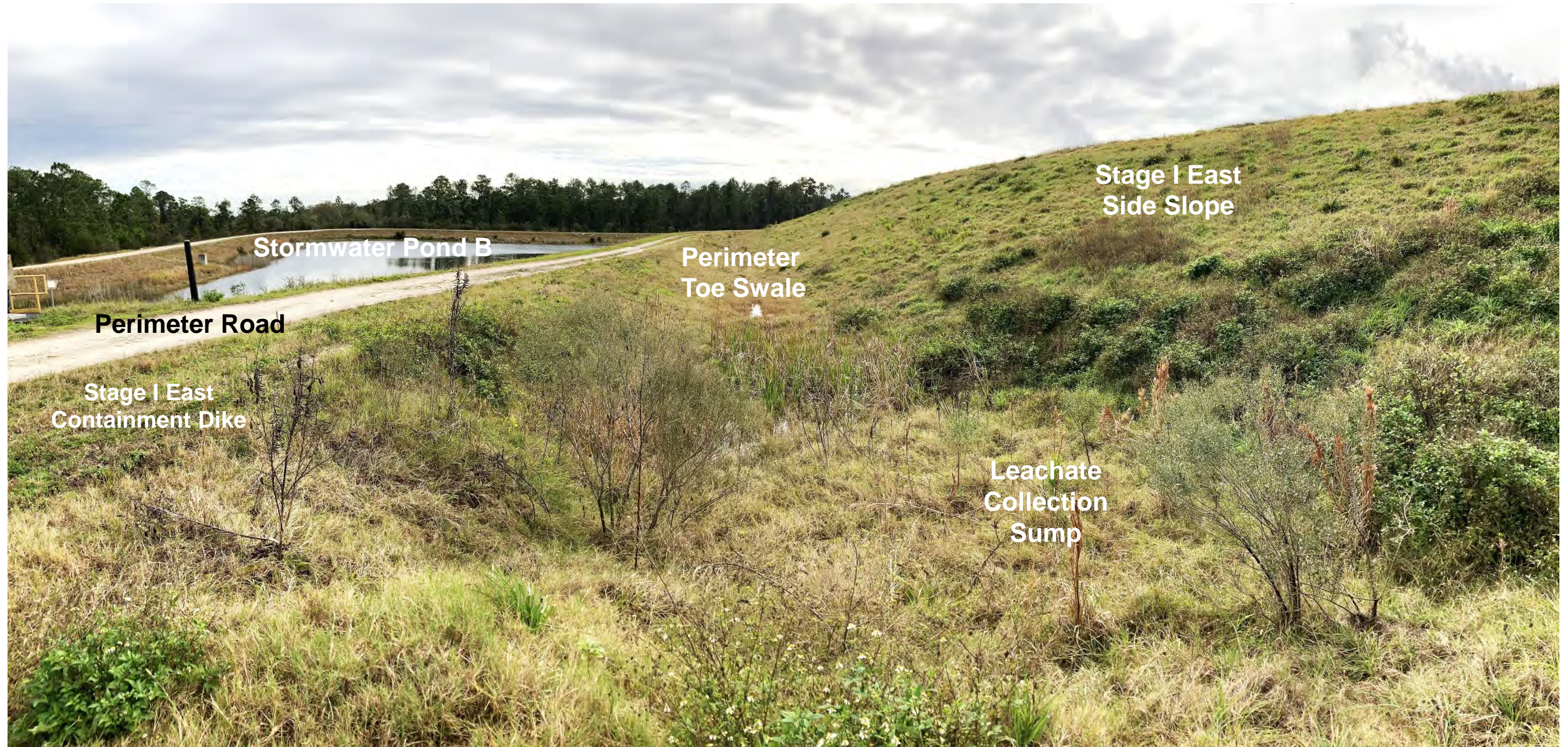
Eastern Side of Increment 1, Stage I, Looking South from Near Leachate Collection Sump
