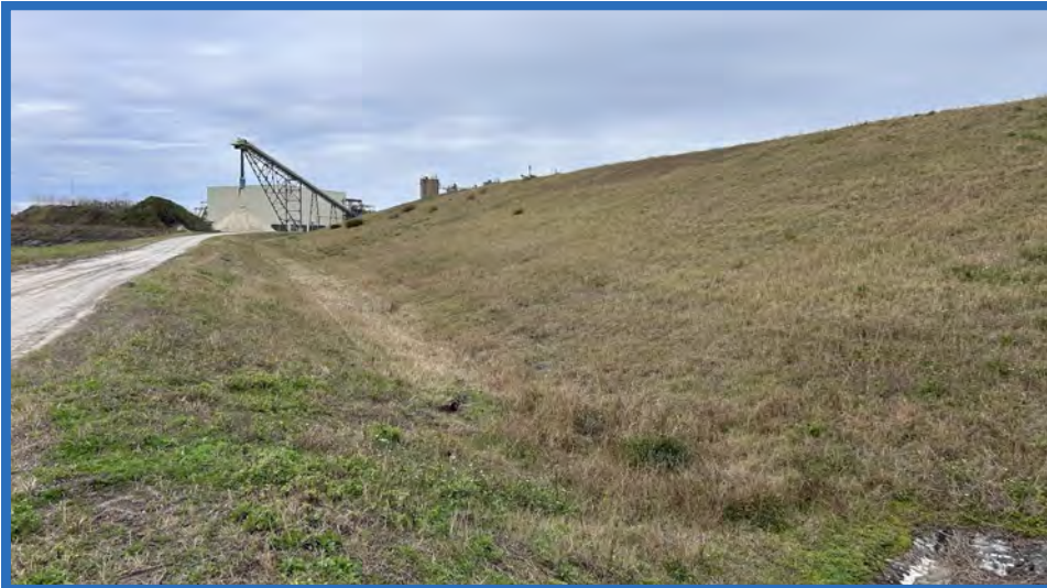
Perimeter Road and Swale South of Increment 1, Looking West; Gypsum Dewatering Building and Silos in EPF Area to Rear of Photo
