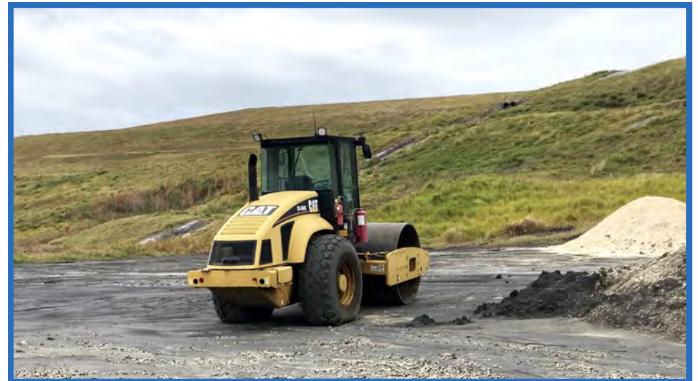
Caterpillar CS-563E Compactor in Stage IIB North of Access Ramp
