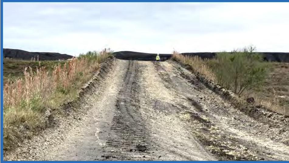
Access Ramp to Stage IIB, Looking East
