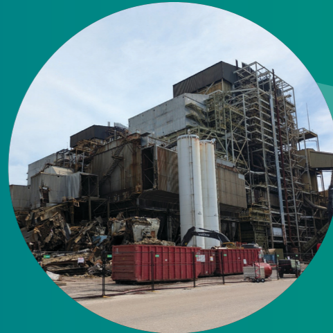
SGS TRANSITION Unit 1 partial demolition begins SGS - Palatka, Florida
